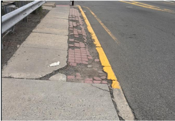
Photo 1 – Anderson Avenue (looking northeast)
